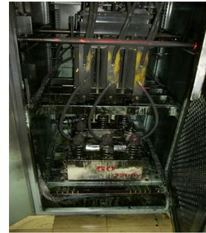
Figure 5. Site of condenser connection fire explosion.
