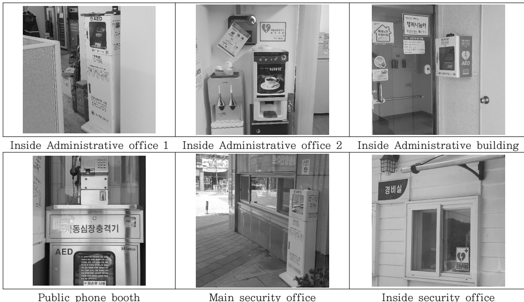
Fig. 1. Installation places of AED.
