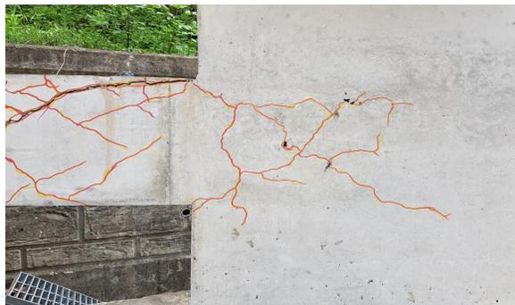
(b) Crack patterns of shear wall
