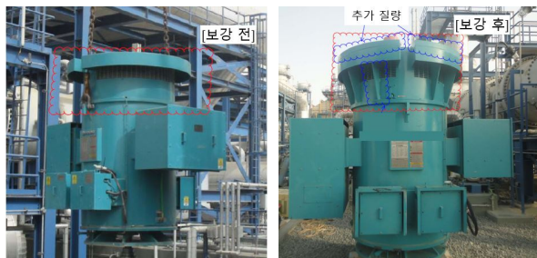
(a) Before retrofitting (b) With added mass
