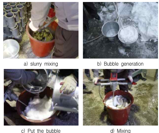
Figure 2. Manufacture of lightweight foamed concrete
