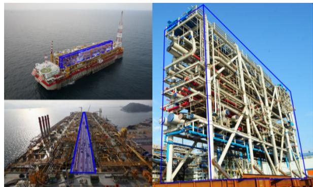
Fig. 4 Example of the pipe rack and the pipe rack module of FPSO
