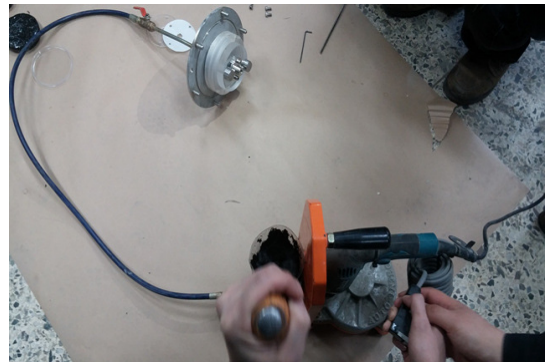
(b) Repair material injection
