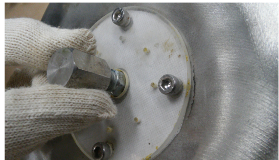
(c) Inlet Bar for injection installation
