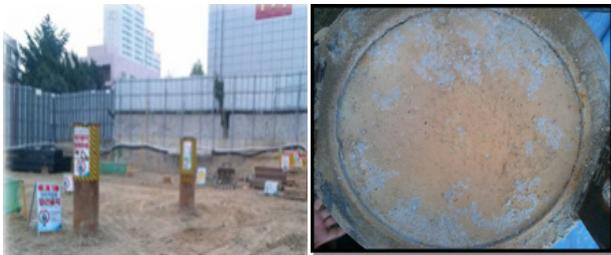
i) Buried CFT steel pipe      ii) CFT steel pipe inside
