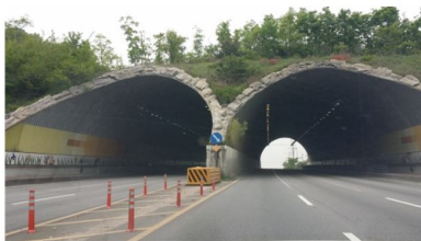
(a) Photograph from road
