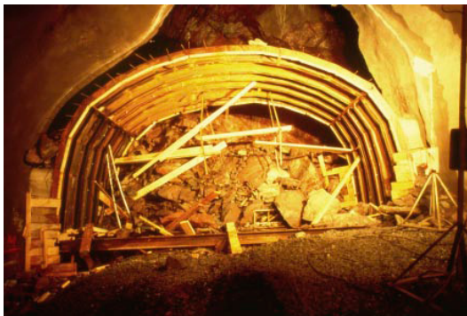
Fig. 8. Overbreak during excavation of Forsmark 3 tunnel (Carlsson and Christiansson, 2007)
