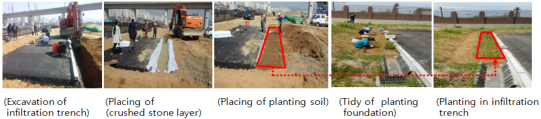
Figure 1. Infiltration trench installation process
