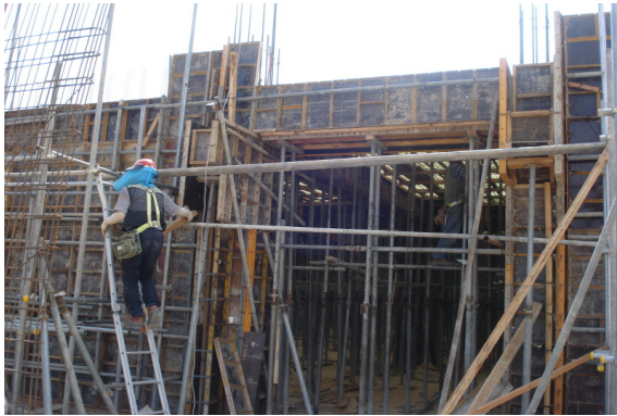
[Figure 4] Uninstallation of temporary staircase
