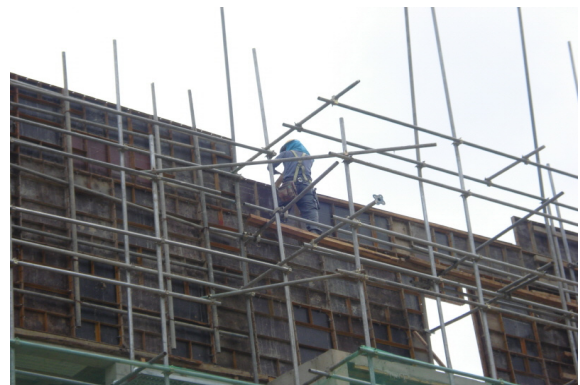
[Figure 3] Uninstallation of walk plate
