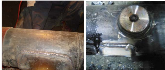
Fig. 5. Examples of the repair using a steel plate patch.
