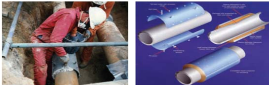
Fig. 1. Epoxy repair sleeve[11].
