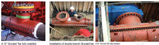
Fig. 2. Repair by grouted Tee[12].
