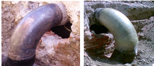
Fig. 6. Composite repair of pipeline elbow.
