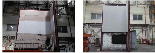
(a) Insulation installation (b) Stone coat finish
