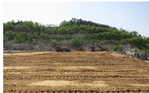
Photo 4. Landscape of the recovering site in the Whaseong quarry.
