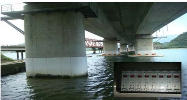
Figure 6: Ti-Mesh anode ICCP system of bridge piles
