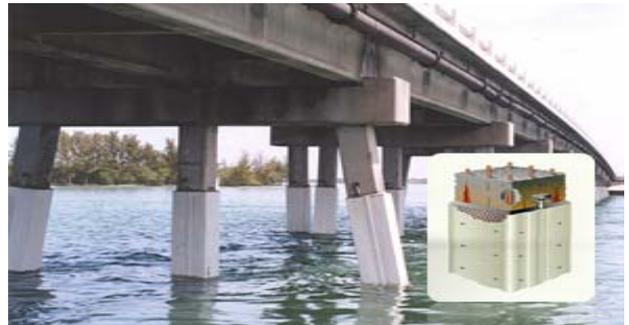
Figure 7: Zn-Mesh anode SACP system in FRP jacket
