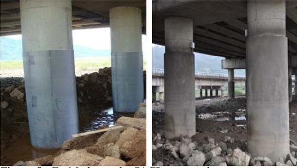
Figure 8: Zn-Mesh anode SACP system in mortar cover of bridge piles
