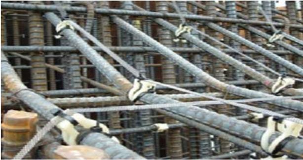
Figure 5: Tied MMO/Ti-Ribbon anode up the rebar
