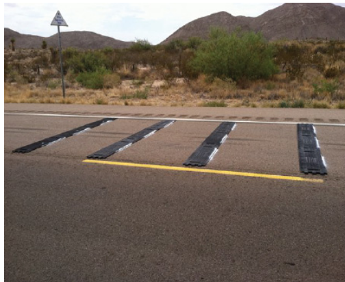
Figure 9. Example of potable rumble strips
