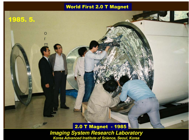
Fig. 2. One of the first 2.0T magnets were installed at Korea Advanced Institute of Science (now KAIST) for research. This is one of the historical event and start producing numerous high resolution anatomical images much superior than the low field resistive MRI of 1.0 K Gauss or 0.1T and opened superconducting MRI era and it remained till beginning of 2000.
