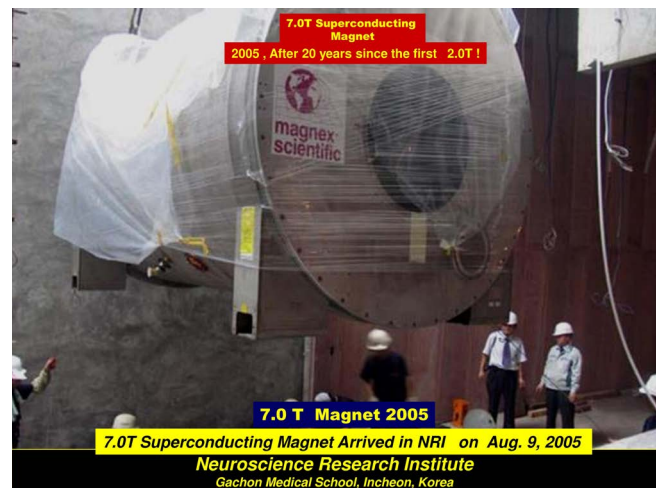
Fig. 3. One of the first 7.0T magnets were installed at Neuroscience Research Institute of Gachon University in Korea in 2005. This prototype required an extensive shielding to protect magnetic field radiation to the external surroundings. Nearly 500 tons of iron sheets were used for the shielding at the time. Today, new self-shielded types became available, therefore, no longer such an expensive and elaborate shielding is necessary.
