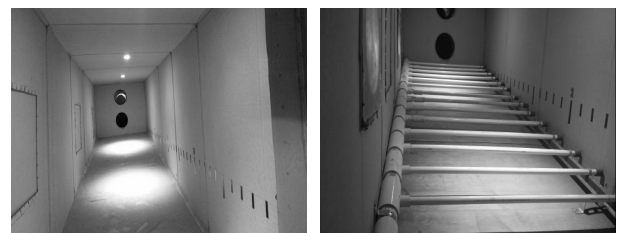
(a) Before install air line (b) After install air line
