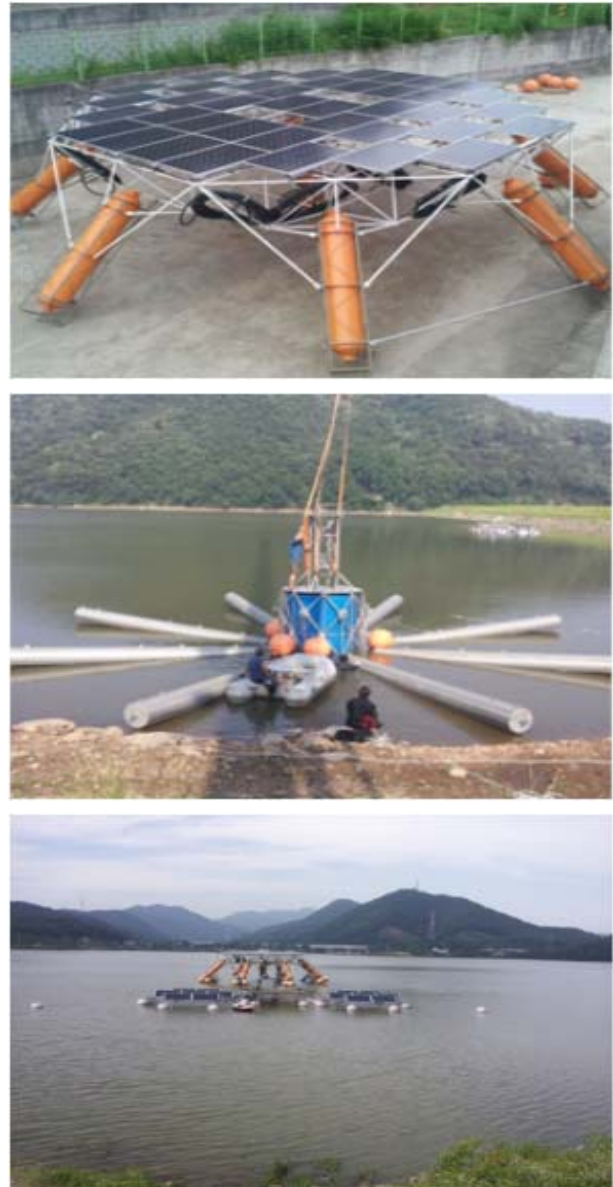
Fig. 5 Production, transportation and installation of floating photovoltaic power generator system
