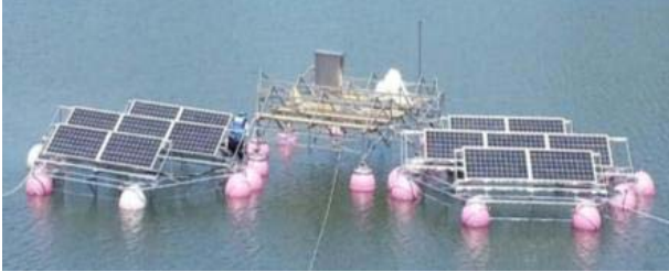
Fig. 11 Fixed type floating photovoltaic system
