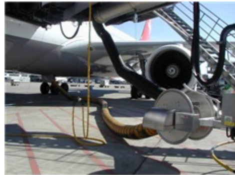
Fig. 9. Fixed ground power systems under bridge [11]
