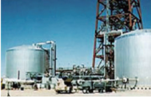
[그림 5] two-tank 시스템(좌 : direct type at the Solar Two power plant, 우 : indirect type for AndaSol-1 and-2) 7)
