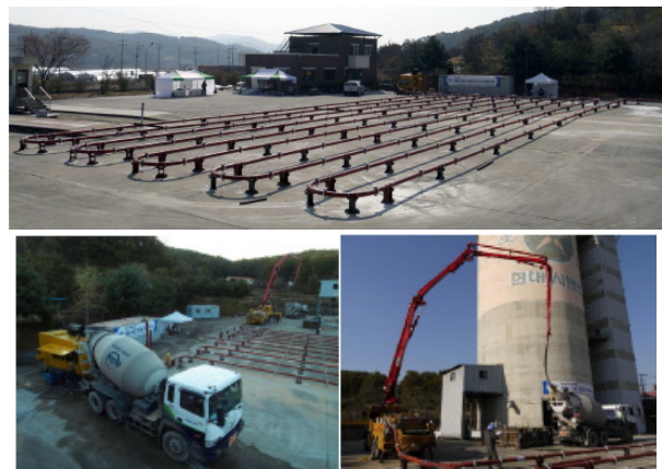
Fig. 2. The whole view of pumping test site
