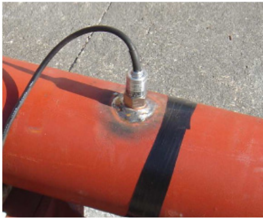
(a) Installation of pressure sensor
