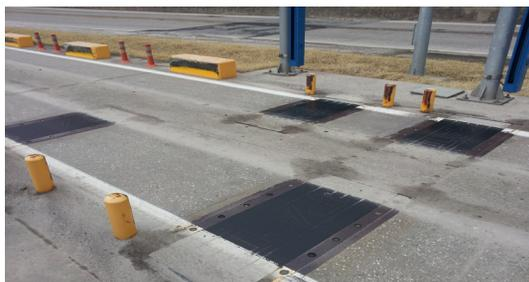
**Fig. 1** Weigh-In-Motion installation for weighing moving truck loads
