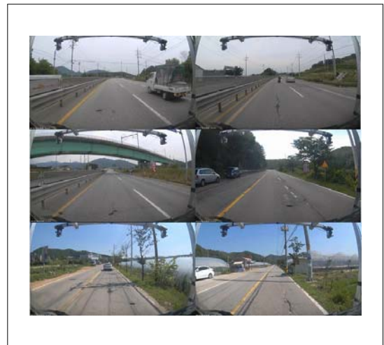
<Fig. 6> Pothole examples
