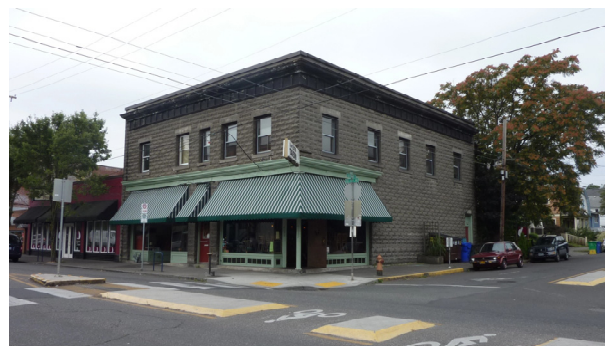
Fig. 1. Typical URM building
