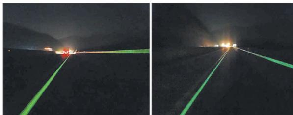
Fig. 2 Test Construction of Luminescent Lanes in Jungbunaeryuk Expressway
