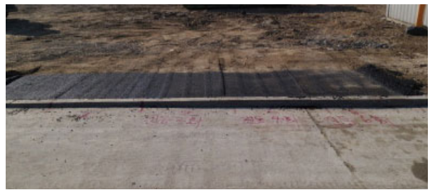
Fig. 5 View of the Testbed after Construction
