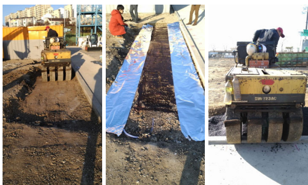
Fig. 4 Construction Process of Testbed
