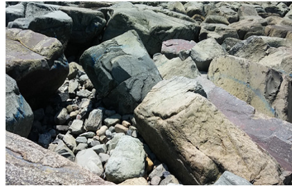
Fig. 8 Deviation of armor stones (Seadike 4)
