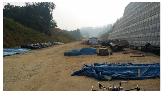
Fig. 6. Testbed Construction Site
