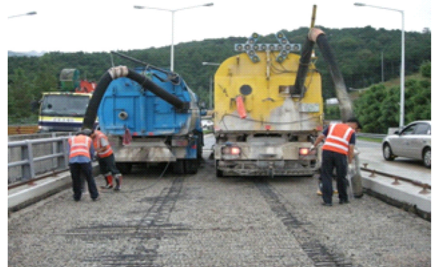
Fig. 5. Bridge Overlay field
