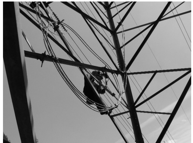
(a) Safety Inspection Scene
