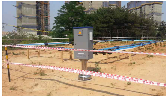
Fig. 11. Picture a test tube, and monitoring systems installation
