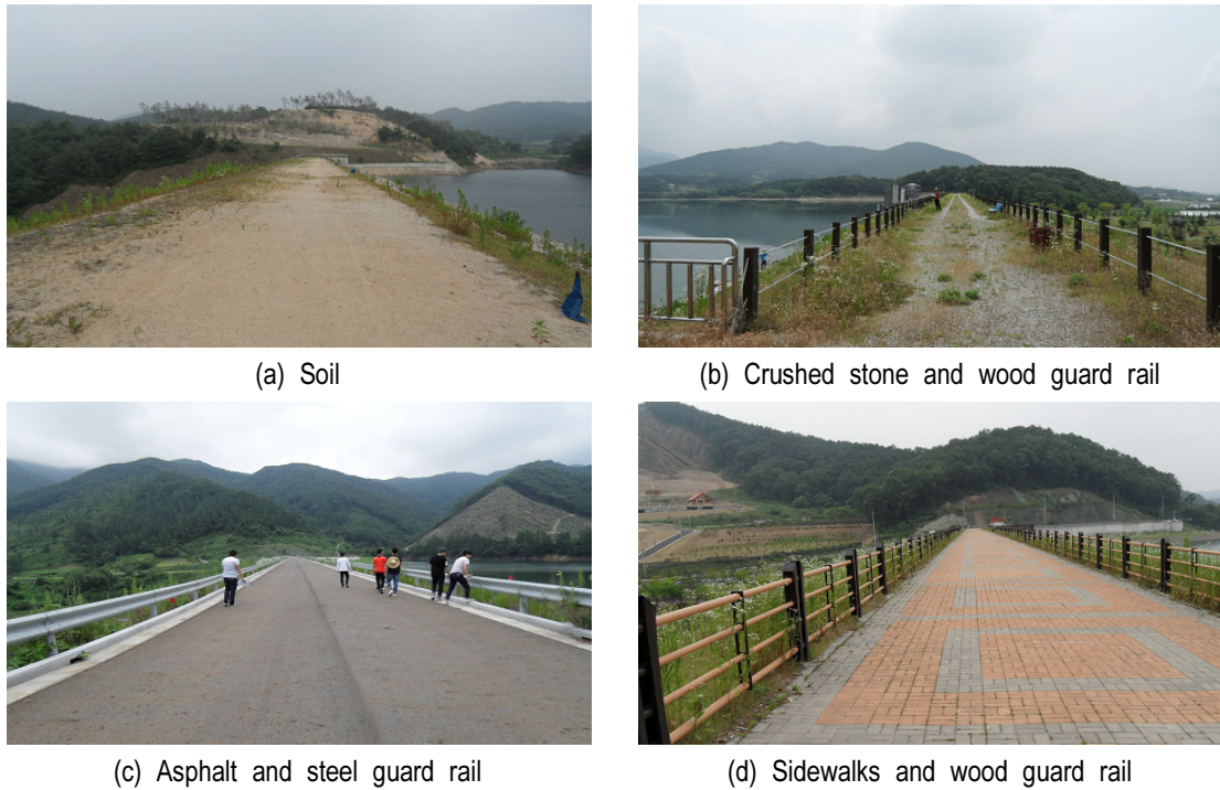
Fig. 2. Shape change and reinforcement of crest.
