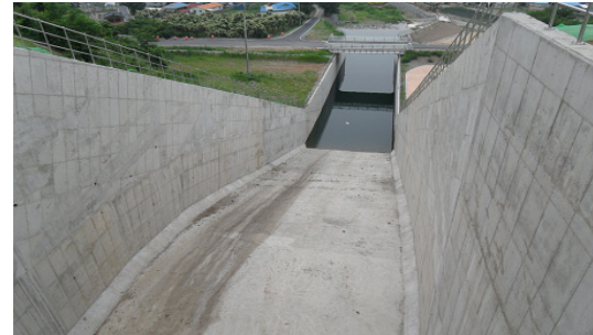
(f) Spillway and hydraulic energy dissipation
