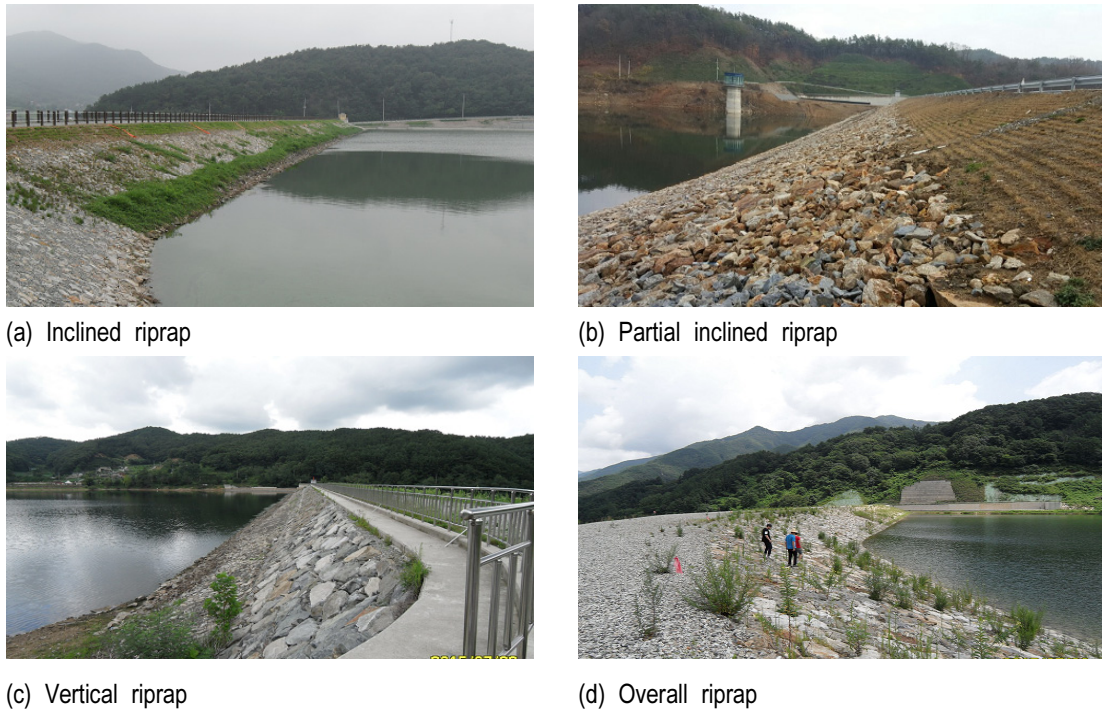
Fig. 3. Shape change and reinforcement of upstream slope.
