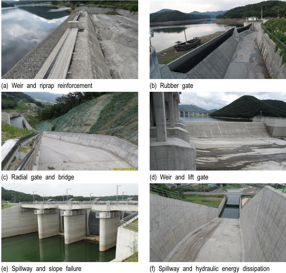
Fig. 5. Shape change and reinforcement of spillway.
