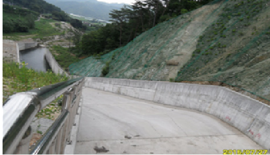
(c) Radial gate and bridge
