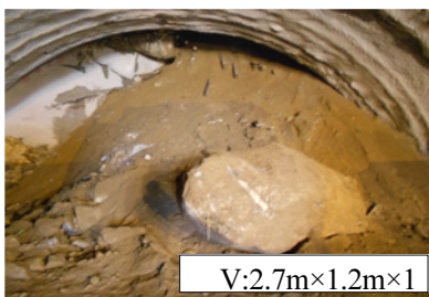
(a) Tunnel face
