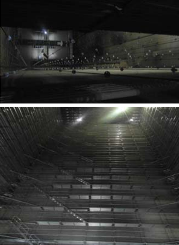
Fig. 6 Application of wire rope type scaffolding system
