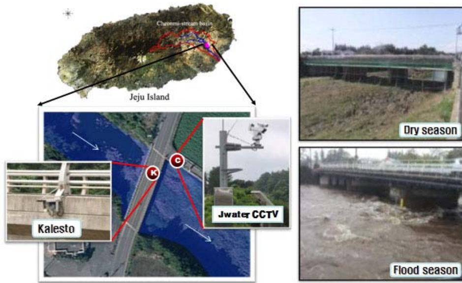
Fig. 2. Location of the Cheon-mi Stream(Observation point: Seong-eup bridge).
