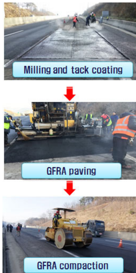
Fig. 9 Construction of GFRA
