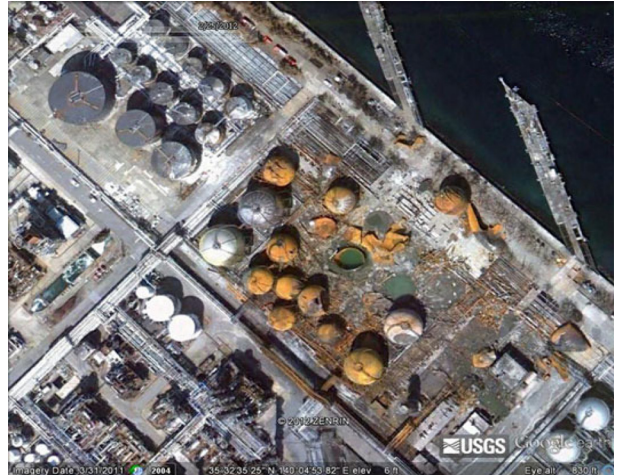
Fig. 3. The LPG tank farm at the Chiba refinery after the earthquake-triggered fires and explosions 13) .
