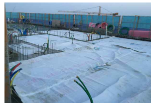
Figure 12. Curing with single-layered white bubble sheet
