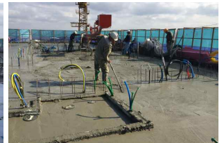
Figure 11. Surface exposure work
