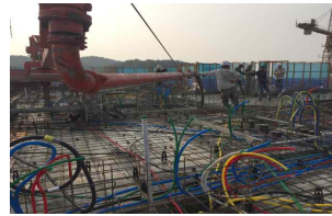
Figure 8. Concrete placement (in progress)
