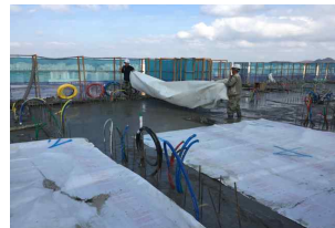
Figure 10. Installation of single-layered white bubble sheet
