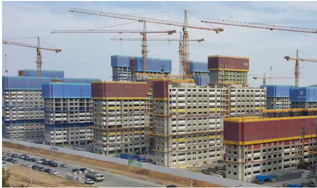
Figure 1. Construction site view
