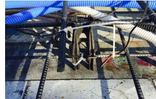
Figure 6. Installation of thermo couple for temperature measurement
