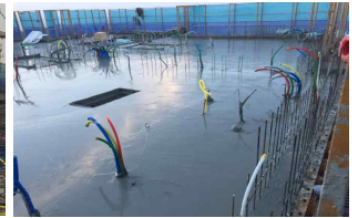
Figure 9. Concrete placement (completed)
