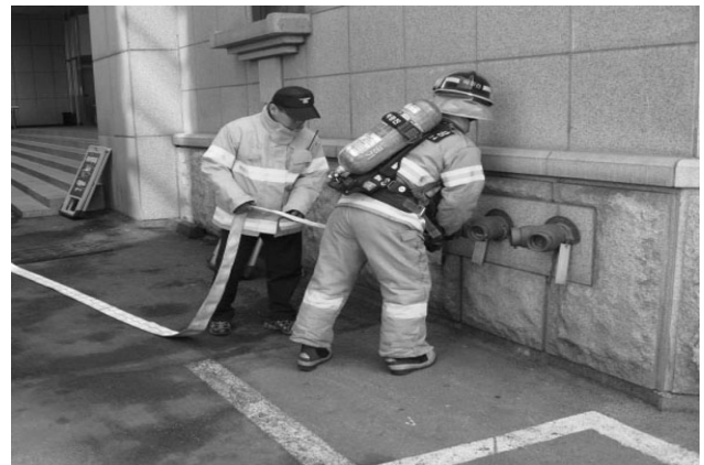
[Figure 2] Fire department connection connecting with water tank fire truck
