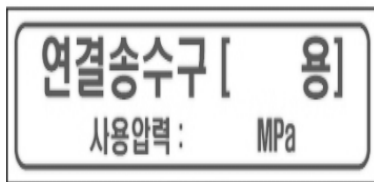
[Figure 5] Pressure sign of the fire department connection
