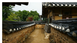
Fig.13. between-yard viewed from the east side inner-gate
