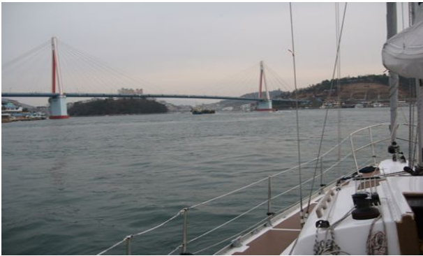
Fig. 5. Passage high of the Dolsan Bridge.
