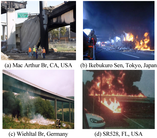
Fig. 2 Bridge fire events caused by underneath fire
