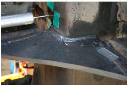
Fig. 11. HBC-1 (cracking at lower diaphragm during 0.05rad)
