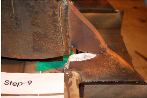
Fig. 14. HBC-4 (failure at lower diaphragm during 0.04rad)
