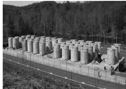
Fig. 1. Dry Storage Facility (Decommissioned Connecticut Yankee NPP).
