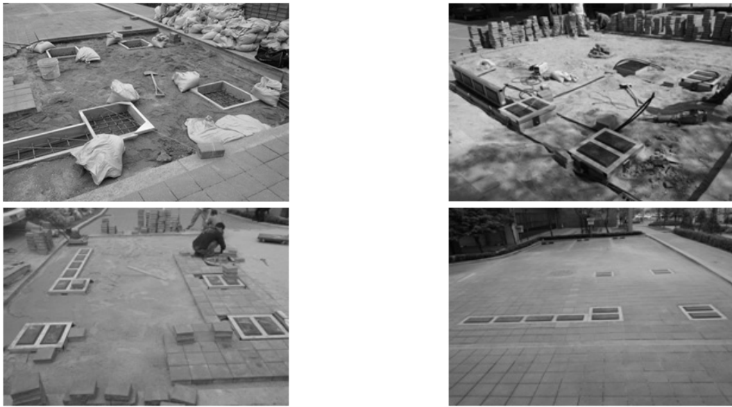
Fig. 12. Field Installation of Improved Energy Blocks Under Passing Vehicle
