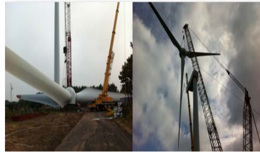
Fig. 2. Wind blade installation processes.
