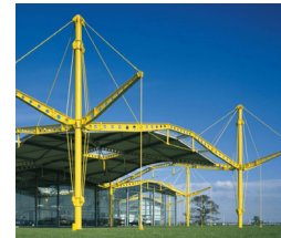
Emphasis on form design attaching angel ties as the stability system
