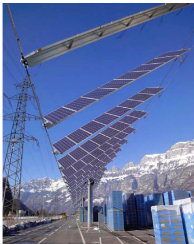
〈Fig. 1〉 Installation of solar wing system 2)
